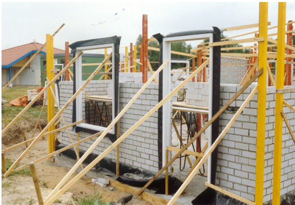
Fenstermontage in den Niederlanden (traditionelle Art)
